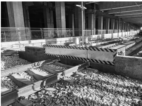
图3 防淹挡板安装现场图 Fig.3 Anti-flood baffle installation picture
