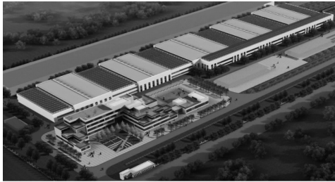
图 1 运用库屋顶分布式光伏发电设施铺设效果图 Fig. 1 Distributed photovoltaic power generation facilities on depot roof
