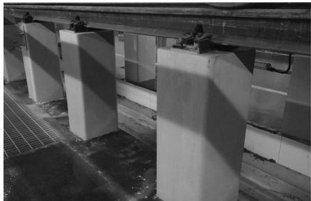
图 8 装配式检修立柱实景 Fig. 8 Real scene of prefabricated maintenance column
